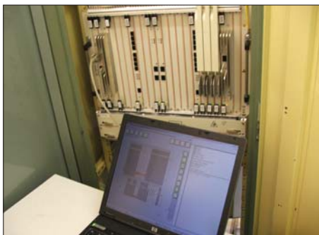
SDH Node Equipment at Otahuhu Substation
